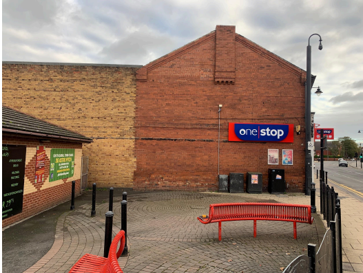
One Stop Shop gable end, Barnsley Road, South Elmsall
