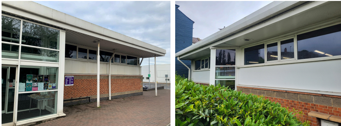
Hemsworth Library exterior [Cladding & windows]
